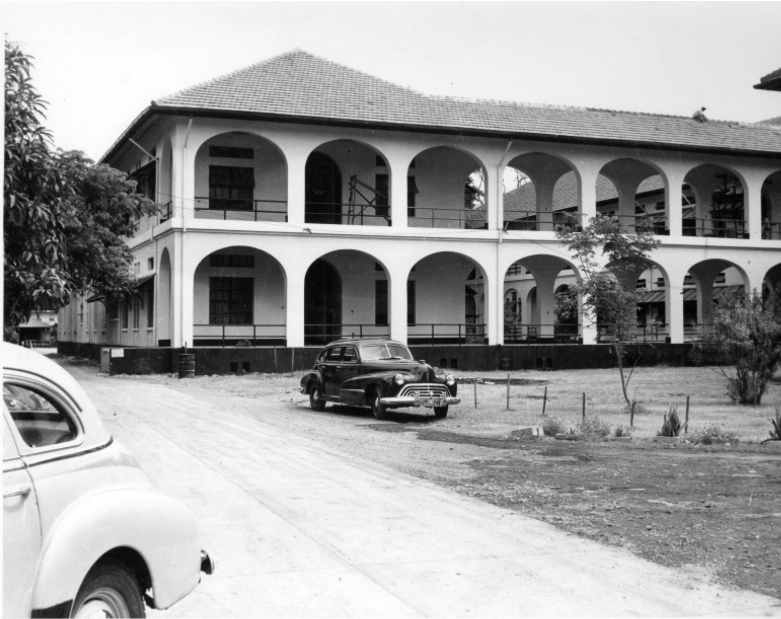
Right Wing of Main Bldg., Phil. Gen. Hospital, Manila
