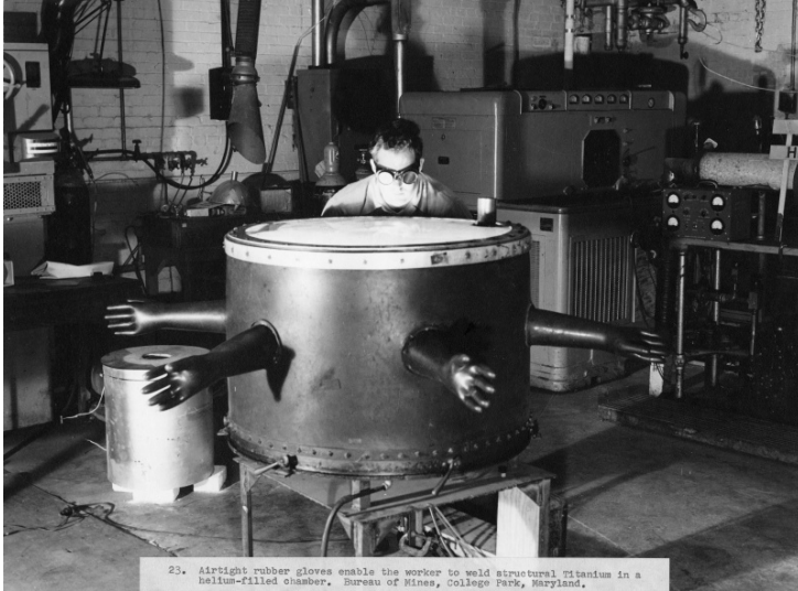
23. Airtight rubber gloves enable the worker to weld structural Titanium in a helium-filled chamber. Bureau of Mines, college Park, Maryland.
