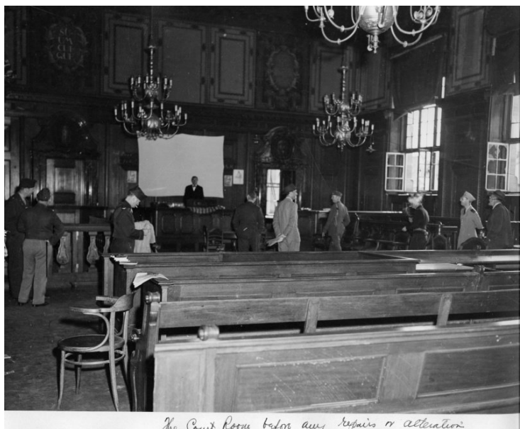
The Court Room before any repairs or alterations
