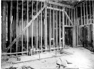
The studding in the White House dating from 1815-1818, in the east wall of Room 14 after the lath and plaster were removed.
